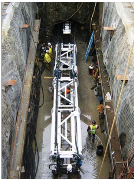
Fox Mill Water Main Project
