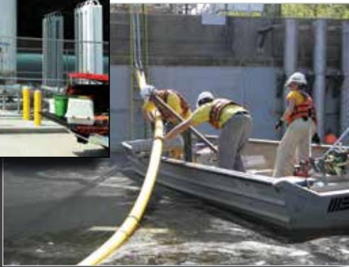
We all know that oxygen is a good thing - right? But did you know that water needs it as much as we do? This past summer Fairfax Water put in place a new system that uses pure oxygen in a unusual way - injecting it into the raw water we draw from the Occoquan Reservoir. The reservoir, along with the Potomac River, provides raw water to Fairfax Water's treatment plants.
